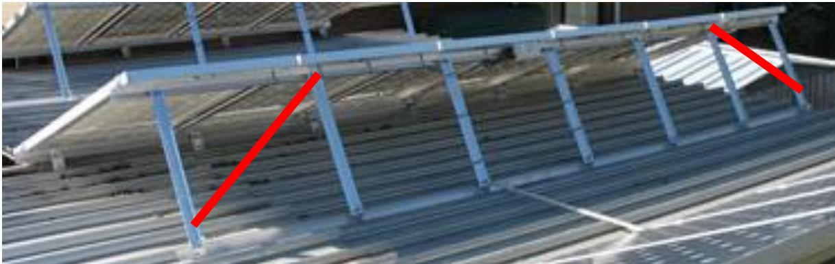
The diagonal brace can cross several tilt legs if required, as shown below:
